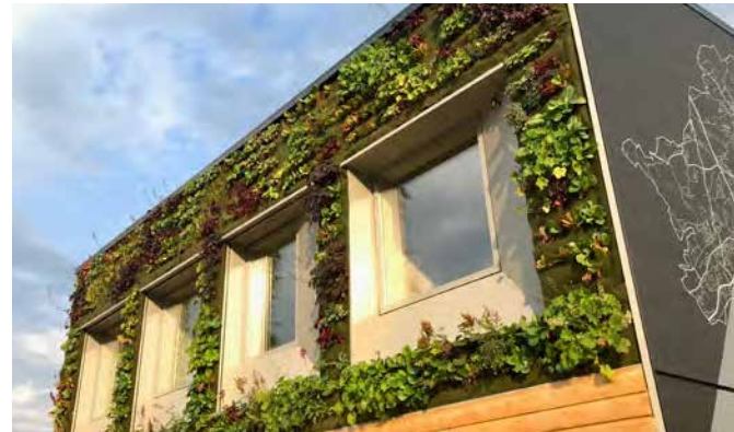
Slanted window reveals increase the incidence of light in the Aachen team's project © SDE 21/22
