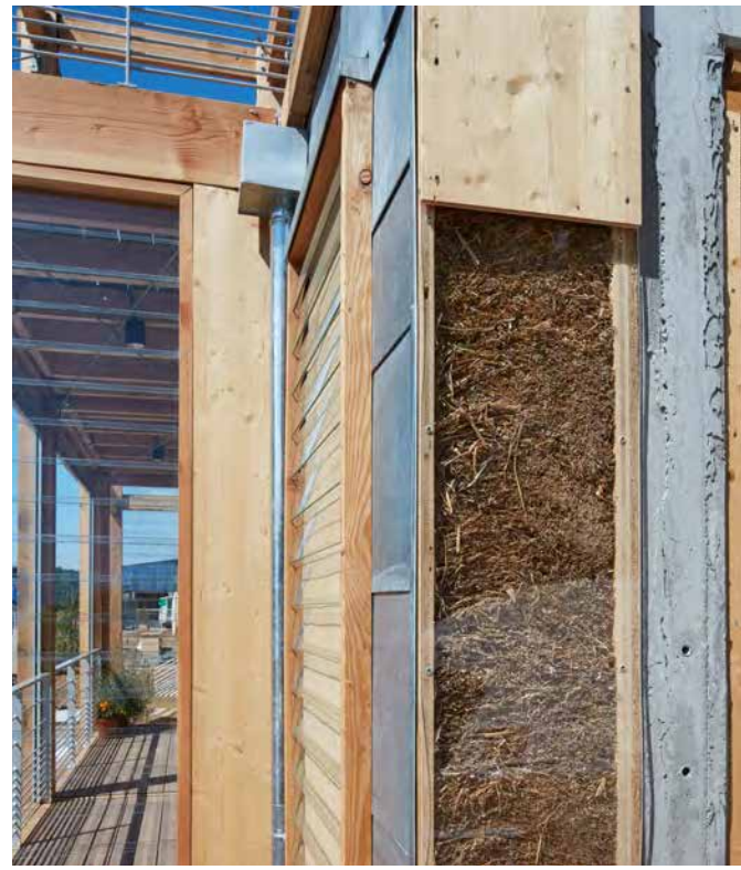
Example of thermal insulation made from renewable raw materials, team Grenoble © Steinprinz / University of Wuppertal
