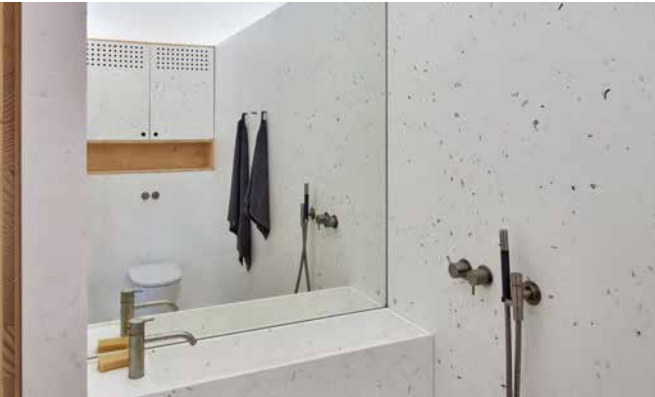
Bathroom surfaces made from recycled yoghurt pot panels by the team from Stuttgart © Steinprinz / University of Wuppertal
