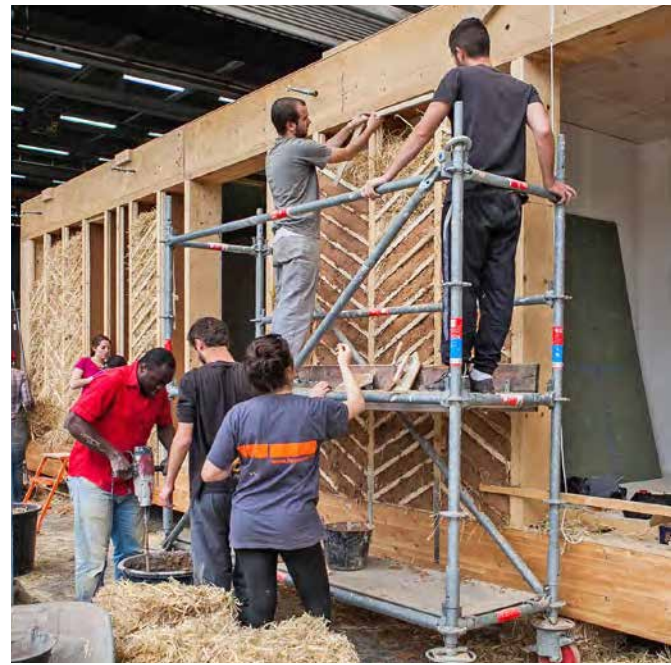
The team from Grenoble is experimenting with straw and clay at “Les Grands Ateliers”. © AuRA / SDE 21/22
