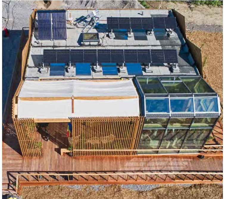
Rooftop with PV modules © Steinprinz / University of Wuppertal
