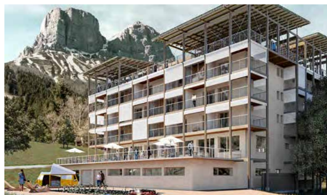
Presentation of the overall design for the transformation of a hotel in the French Alps near Grenoble. The transformation contributes to using the load-bearing components for a long time © Team AuRA / SDE 21/22
