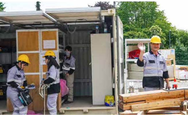
Extendible and retractable solar modules on the tool container to provide construction electricity for the team from Taipei © SDE 21/22
