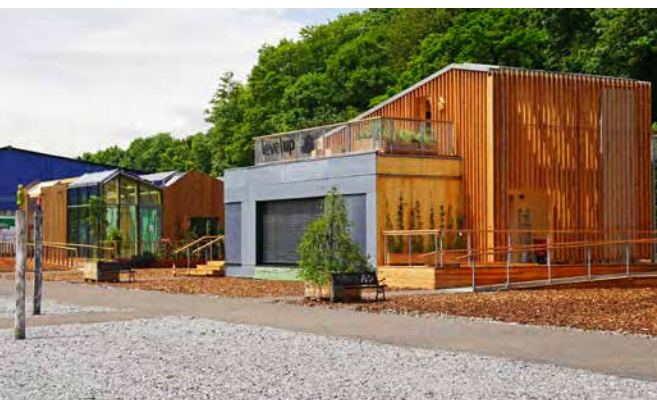
Preparations for the garden landscaping and the finished site
